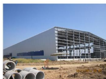
Figure 11: New automated precast factory to start operations in Mar 2012
