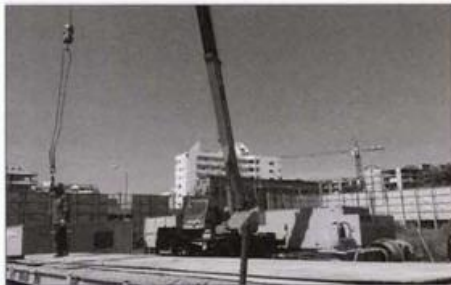
Piling work for the project gets underway on Soi 5, Pratumnak Hill.
